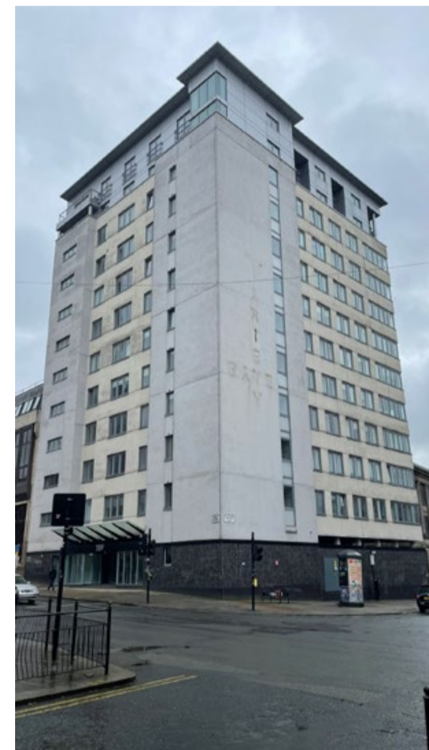
Site of Former Renfield Church. Demolished 1964
